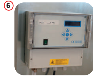
6 CYCLIC PROGRAMMER WITH PRESSURE DROP CONTROL (PLC): a sealed container is used with a transparent lid, duration of injection and pause phases are preset but easily changeable.
